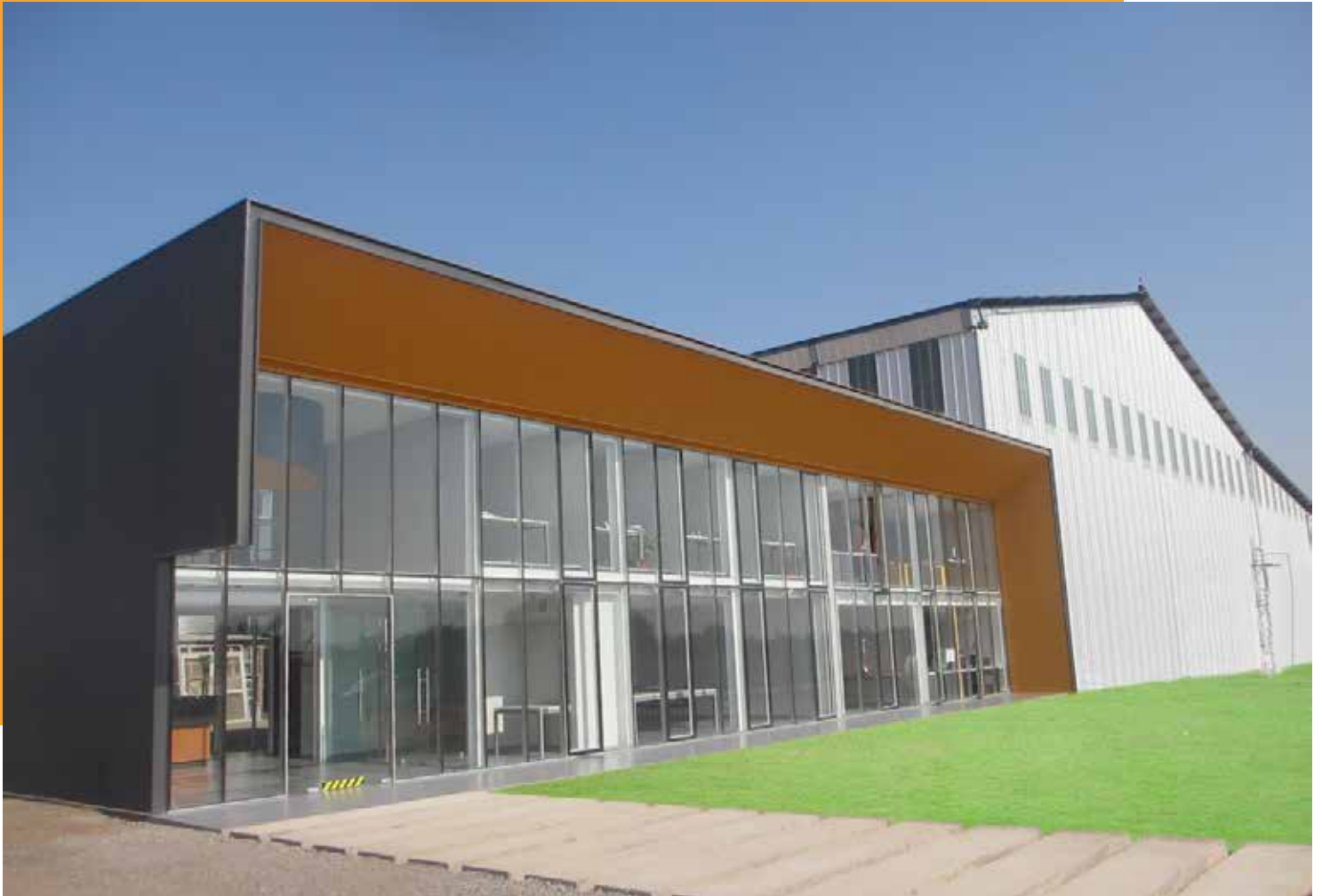
Foto 1.1 Planta KRAH® PIPING SOLUTIONS
